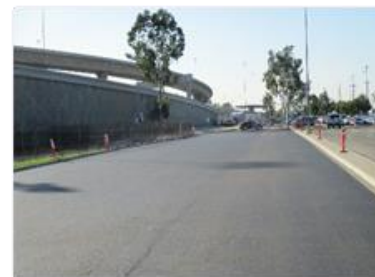
FPNR Asphalt Pavement Replacement
