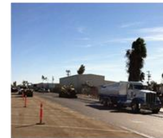
GG Asphalt Pavement Overlay
